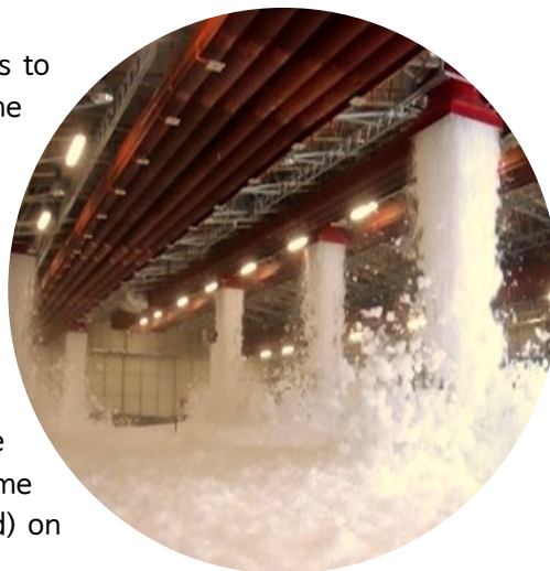
Fig. 3 Fixed foam fire-extinguishing system
